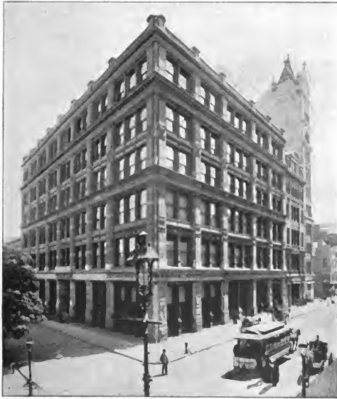
W. & J. SLOANE, BROADWAY, SOUTHEAST CORNER 19TH STREET.
